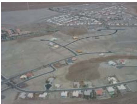
As development occurs in Bullhead City, areas of level terrain, like that pictured here, are becoming scarce.
