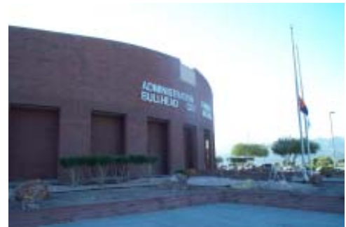
The area of the Bullhead City Administration Complex has become a center for civic, recreation, retail and employment activities.
