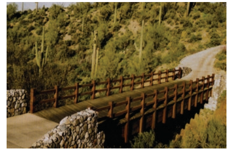
Building bridges to allow for natural flow of water, growth of vegetation and movement of wildlife.
