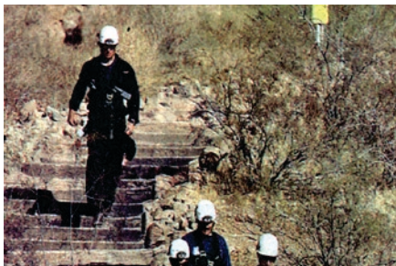
Providing a safe and stable trail treatment over steep slopes for easier accessibility.
